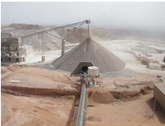
Crushed stockpile cone and conveyor to mill, ROM pad in background
