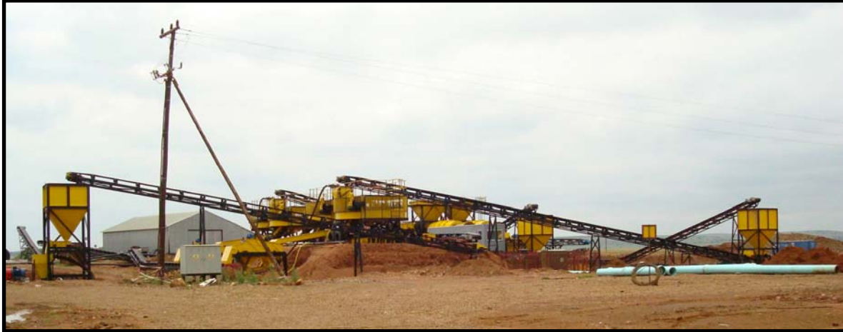
Installation of new plant facilities at the Tirisano mine site
