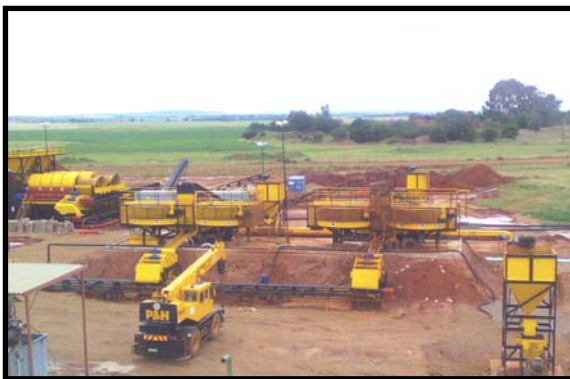
Installation of four sixteen foot pan plants
