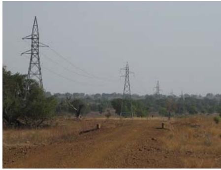
Lattice towers erected on the Ghana side of the powerline route
